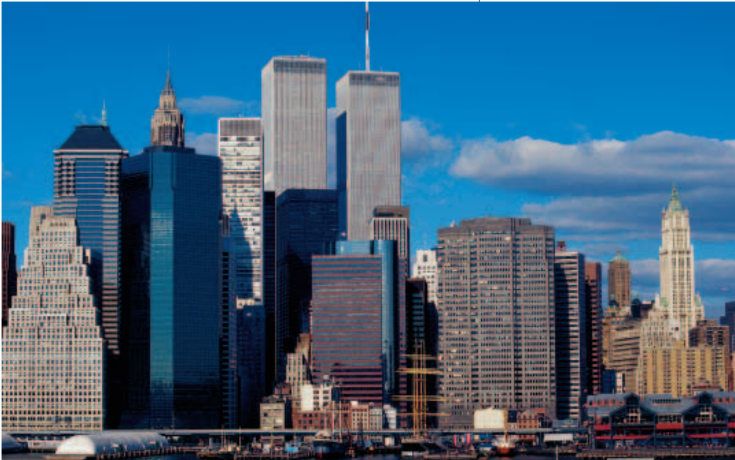
On September 11, 2001, terrorists crashed two planes into the twin towers of New York City's World Trade Center (two tallest buildings in center of photo), causing both to collapse.
